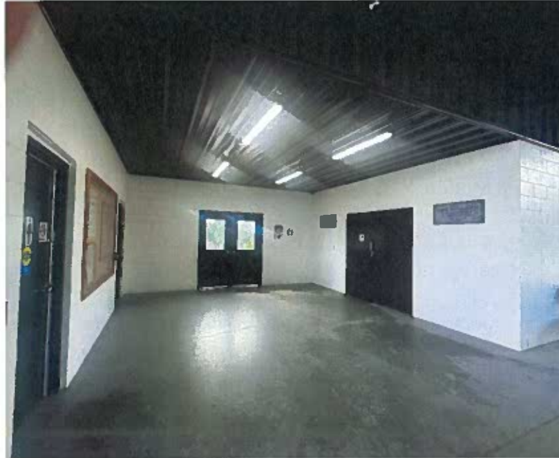
Above: All three white brick walls in the interior
