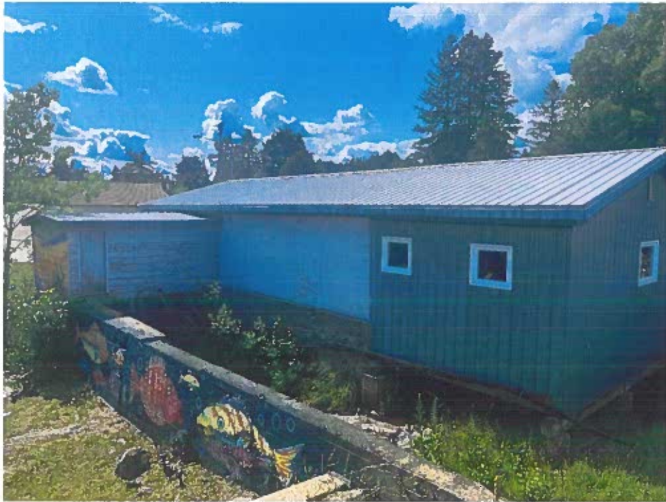
Above: Long Wall with Two Windows
