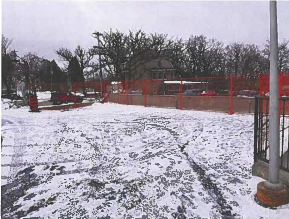
View of a new retaining wall alongside a gravel-filled parking lot.
