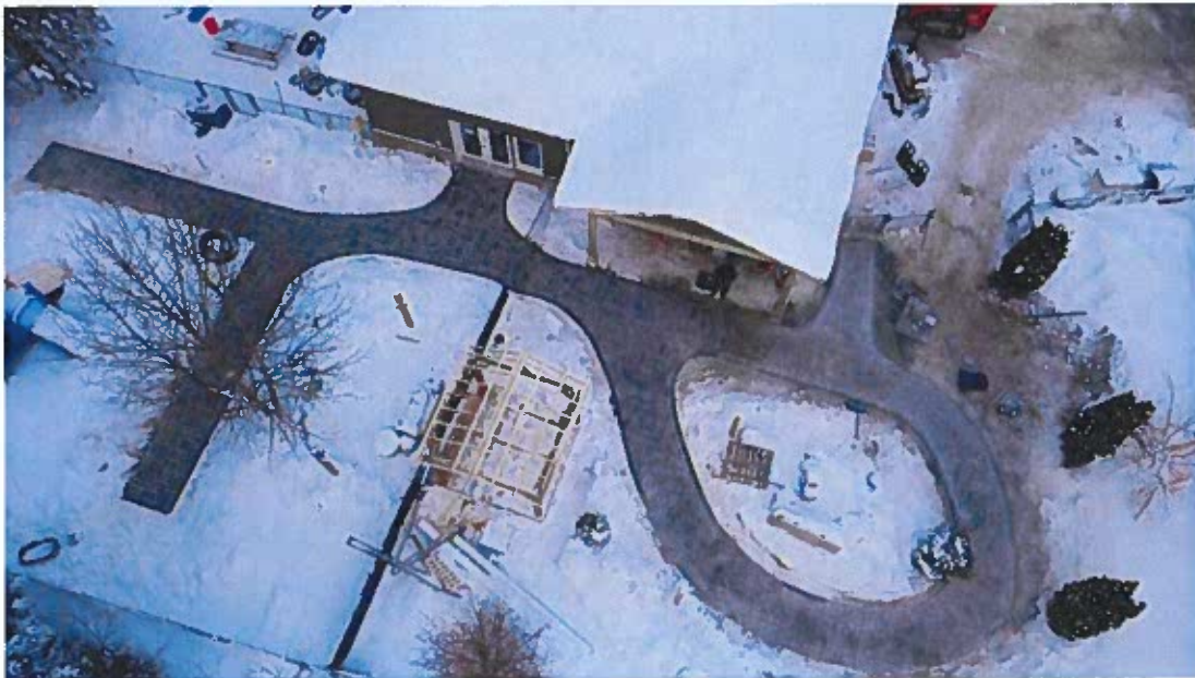
View of new permeable paving installed at a daycare facility.
