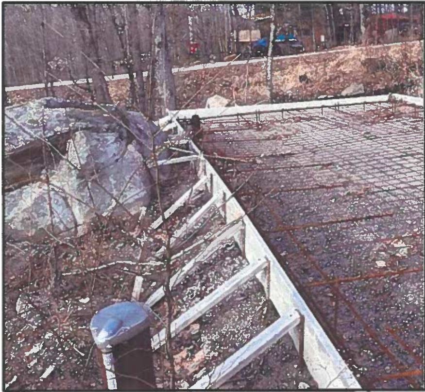
Slab form facing Magnet Road
