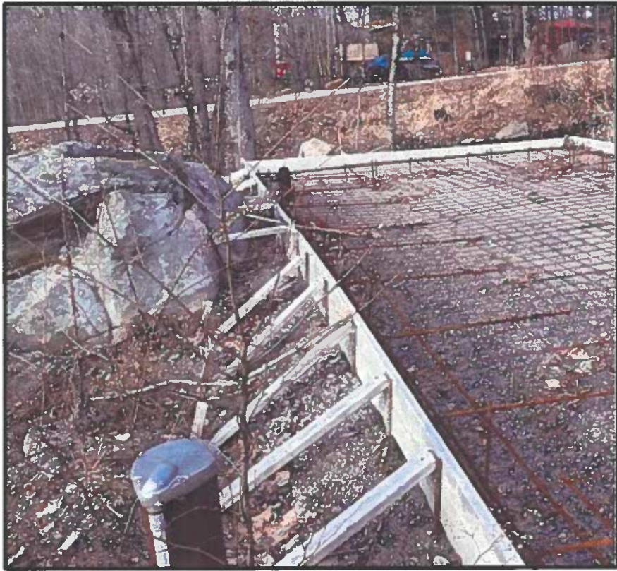
Slab form facing Magnet Road
