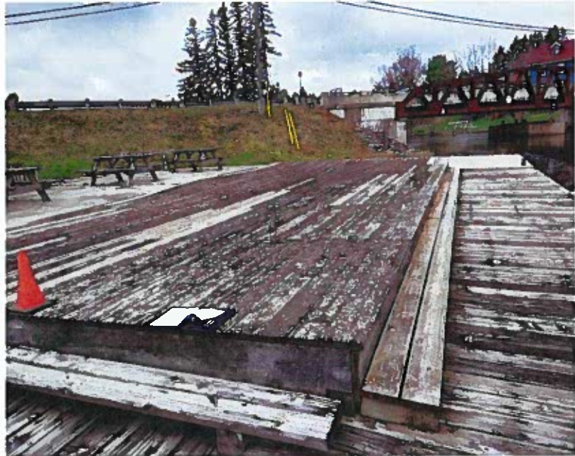
Upper deck area showing general poor condition of decking and uneven surfaces adjacent to the concrete patio
