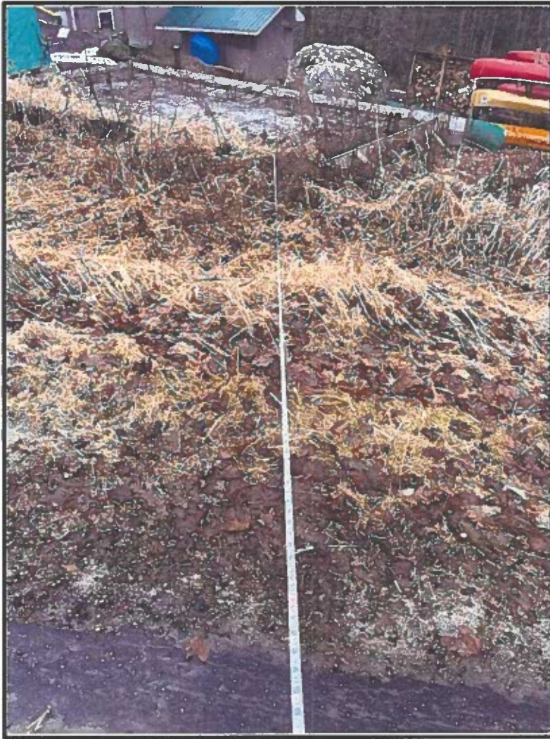
Road pavement facing property
