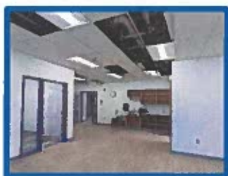
Entry from hallway/office
