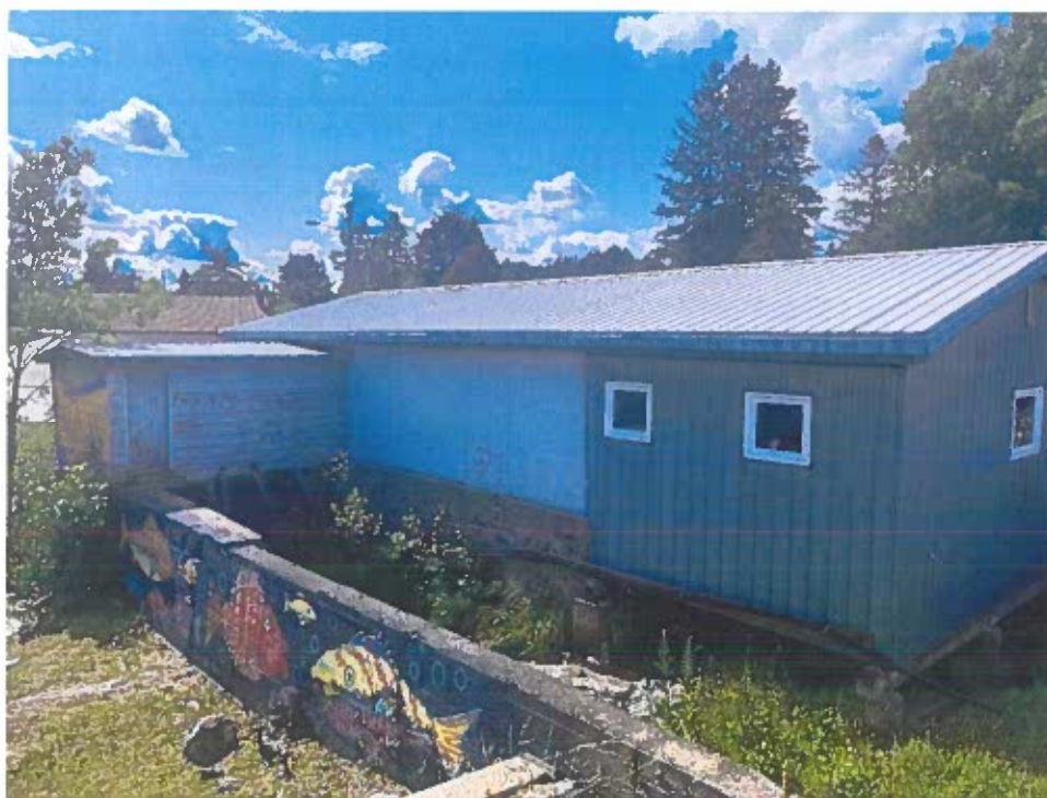
Above: Long Wall with Two Windows
