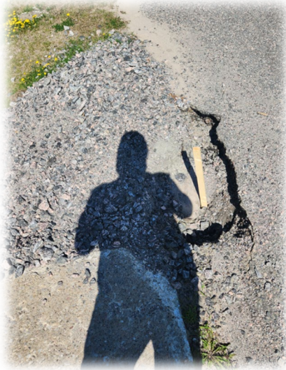
Figure 3: 47'' Sink Hole – West Abutment Figure 4: Approx 12'' Sinkhole – East Abutment
