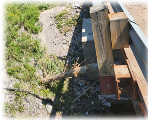
Figure 2: Erosion West abutment
