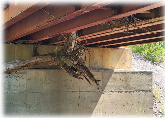
Figure 1: Debris in underside
