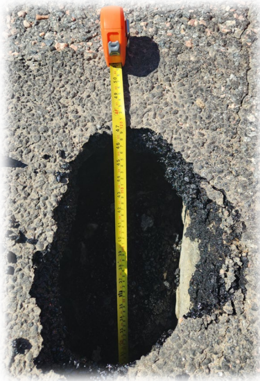
Figure 3: 47'' Sink Hole – West Abutment Figure 4: Approx 12'' Sinkhole – East Abutment
