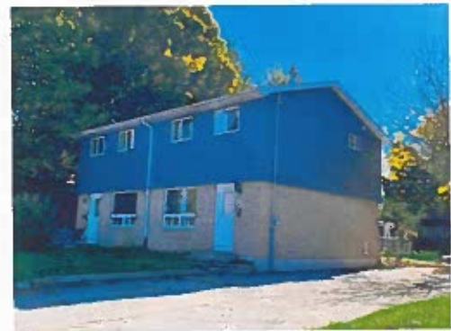
View of a completed siding replacement project
