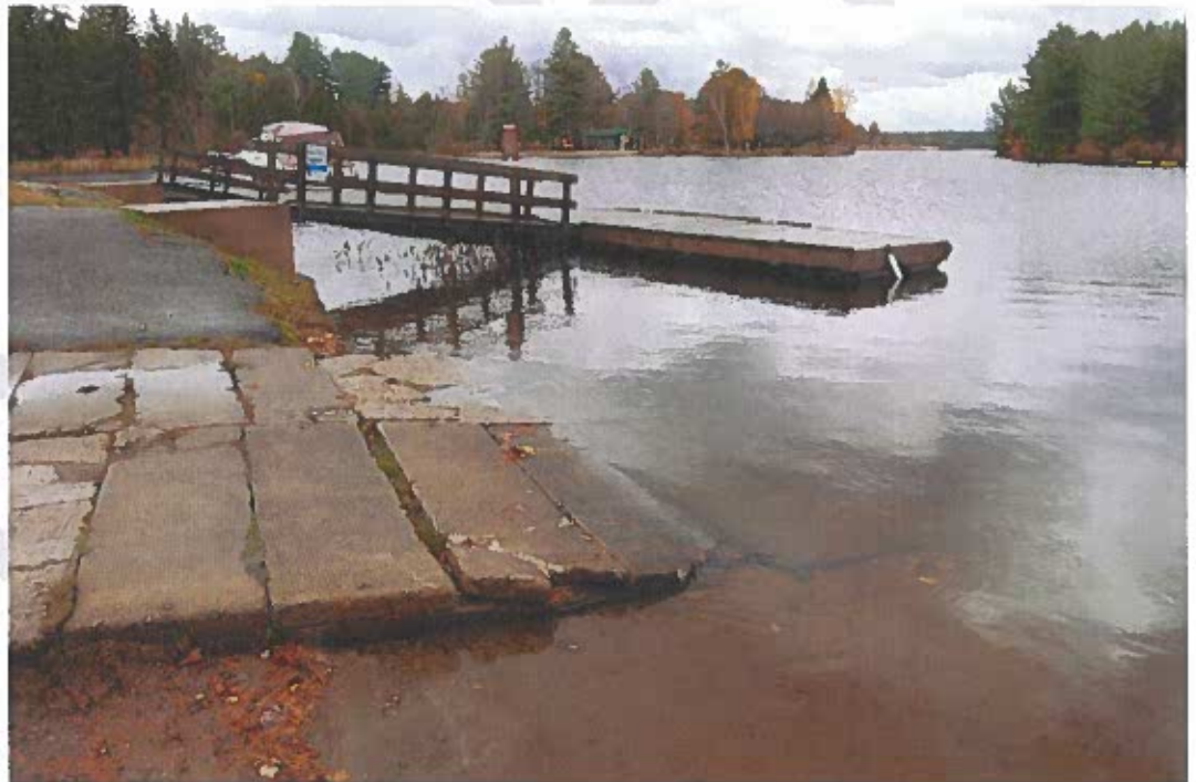
General view of ramp showing condition of slabs above water
