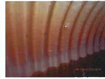
North Wall at Midspan Barrel
