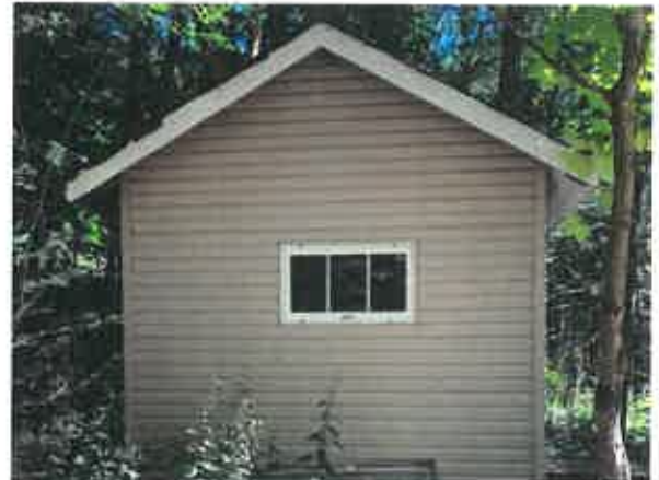
Utility shed 10' by 12' - white square
