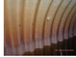
North Wall at Midspan Barrel
