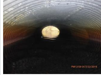
Looking East through Barrel
