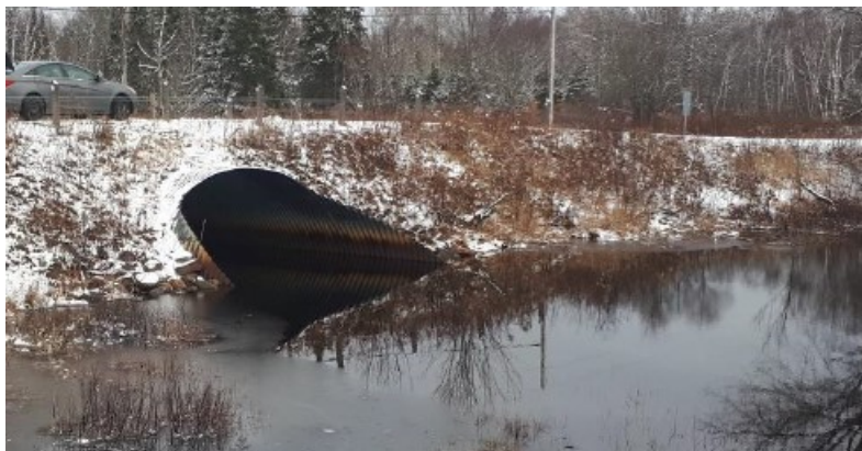
Figure 4 – Existing CSP Elliptical Culvert
