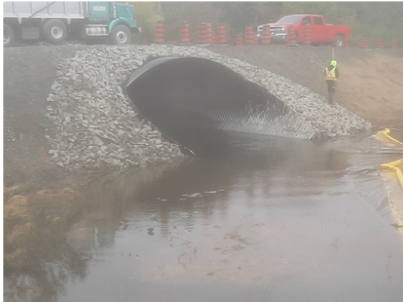
Figure 5 – New Polymer-Coated CSP Ellipse Culvert
