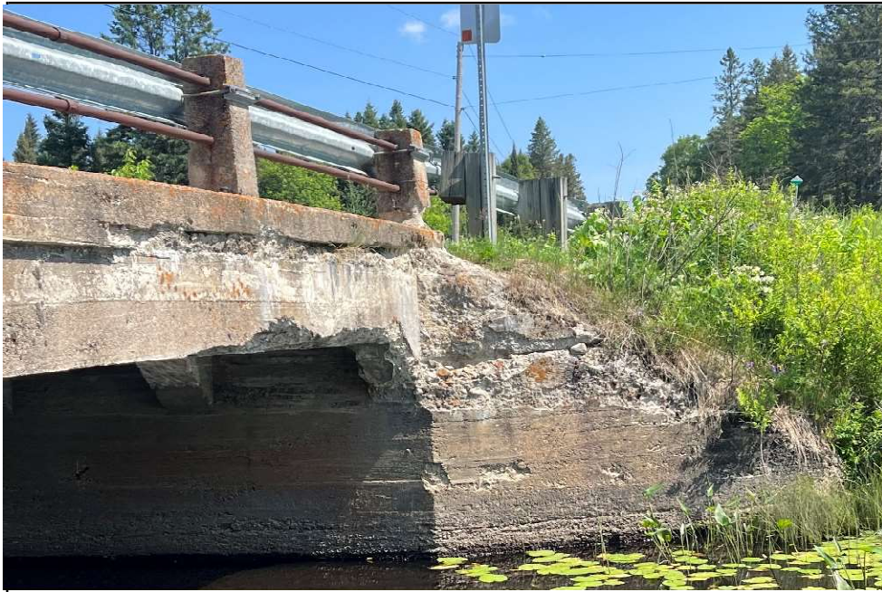
Photo 5: Typical Wing Wall
