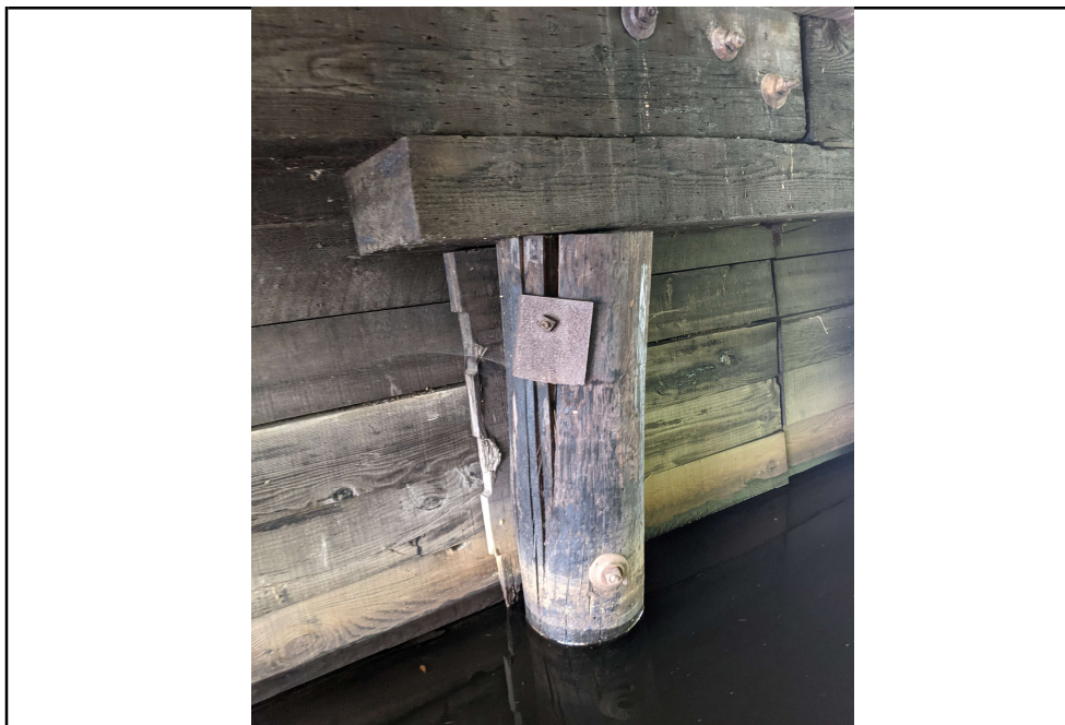
Photo 2: Failing Pile
