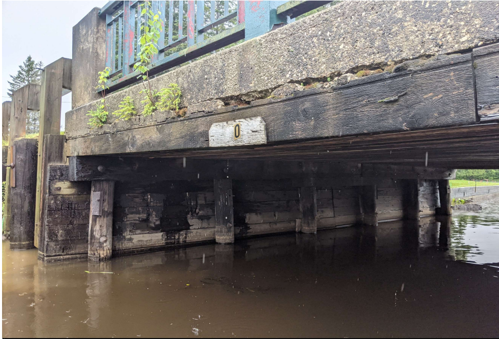
Photo 1: Damaged Soffit And Piles
