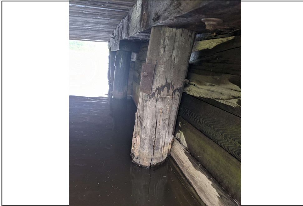
Photo 3: Failing Pile
