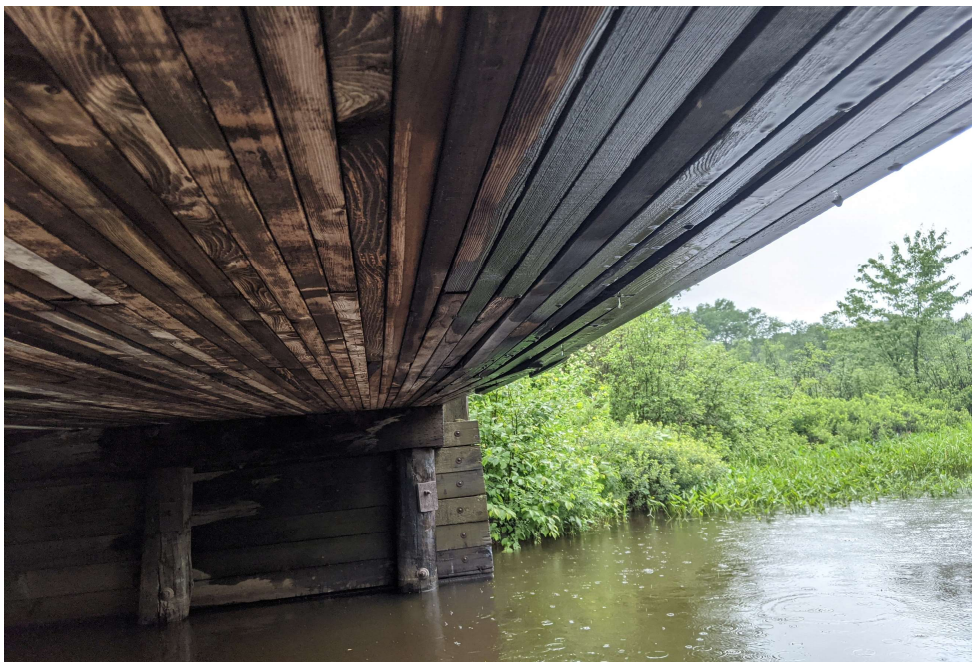
Photo 4: Sagging of Soffit
