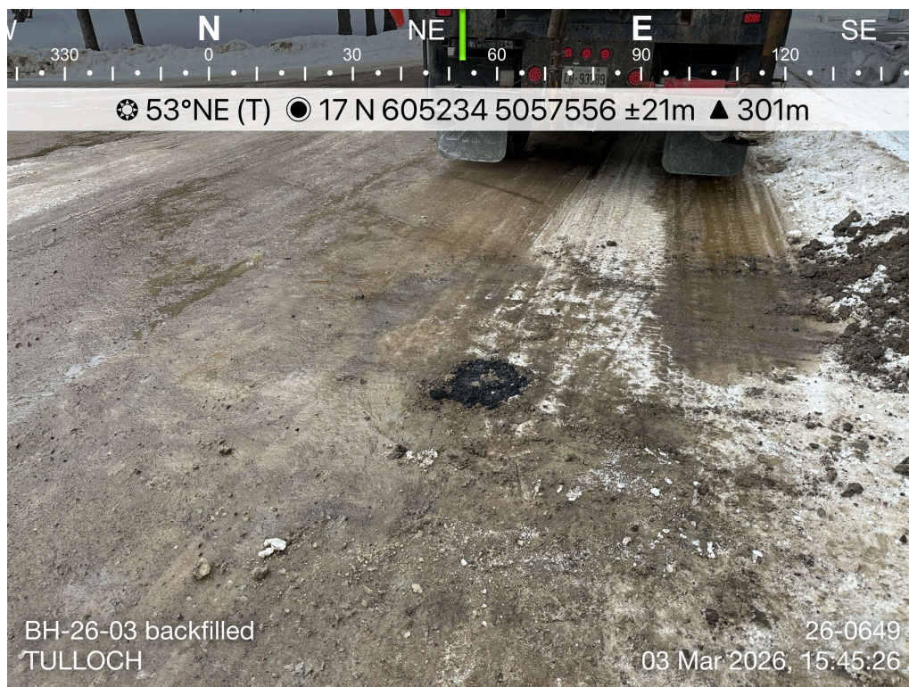
Photo 10: BH-26-03 backfilled. Photo taken facing northeast.
