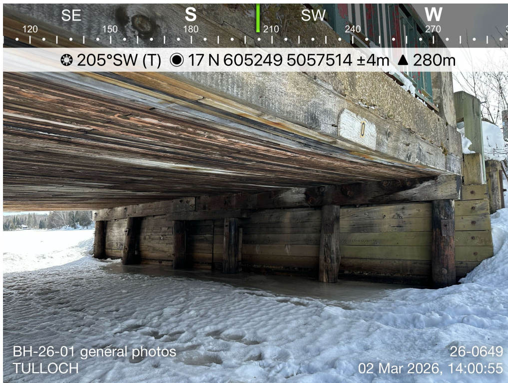
Photo 4: Existing Bridge – West Abutment.
