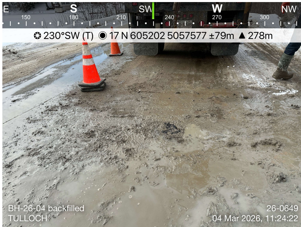
Photo 12: BH-26-04 backfilled. Photo taken facing southwest.
