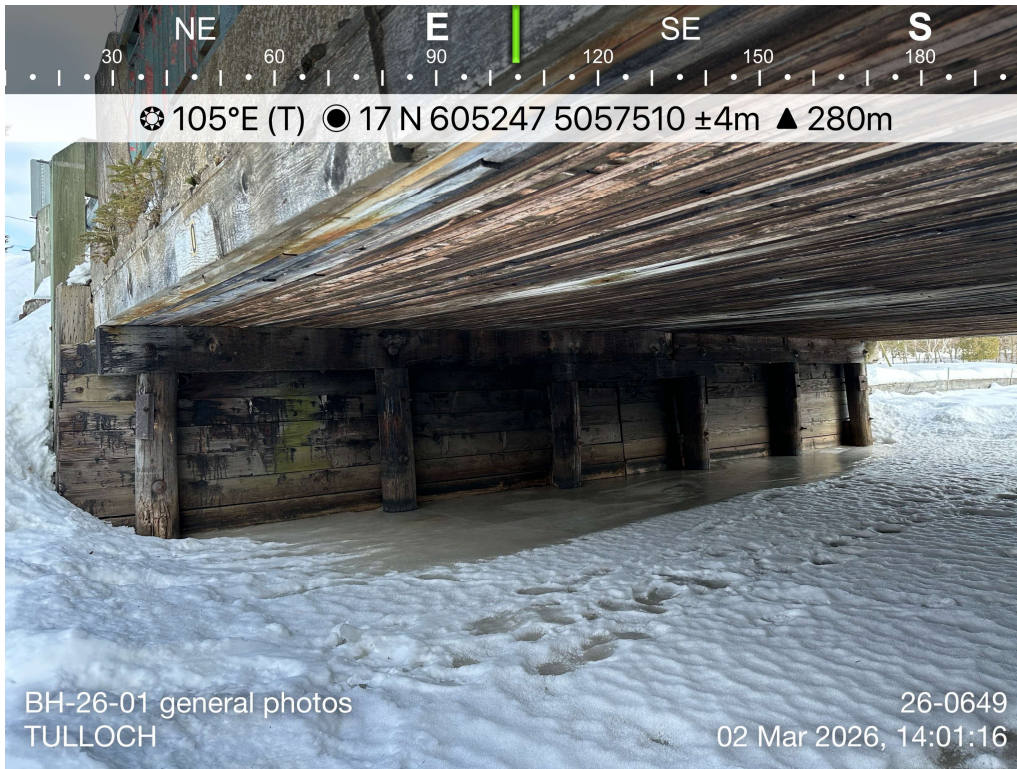
Photo 3: Existing Bridge – East Abutment.
