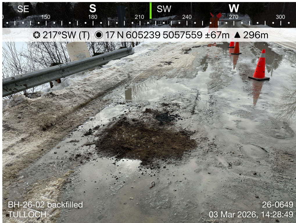
Photo 8: BH-26-02 backfilled. Photo taken facing southwest.
