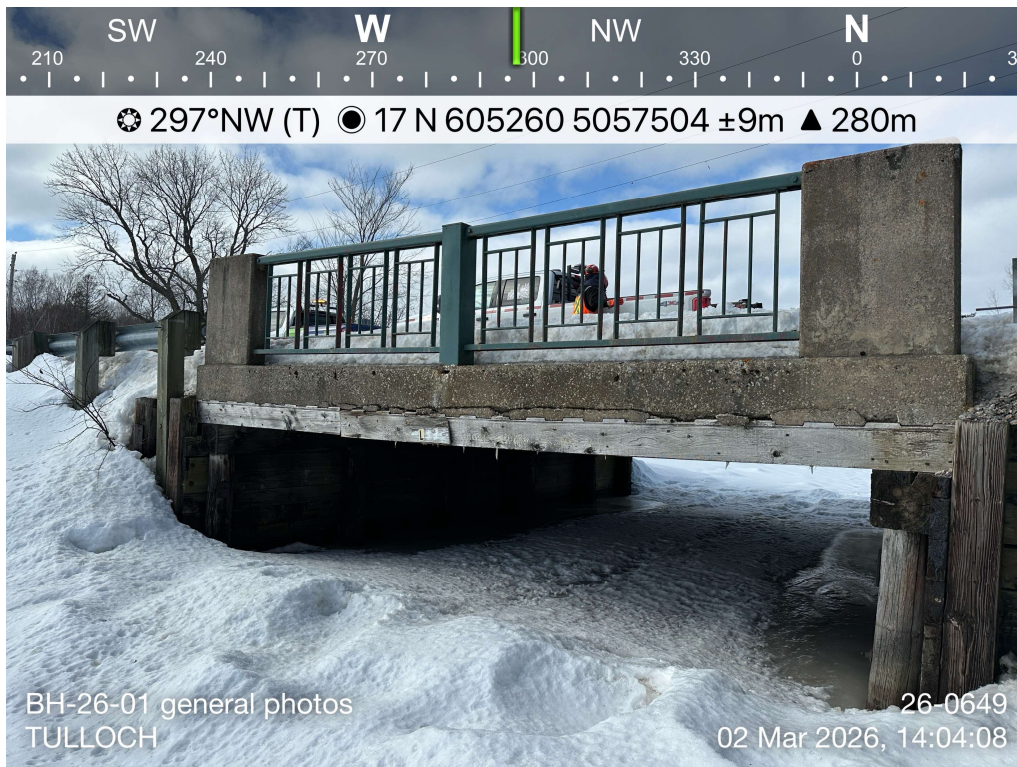
Photo 2: Existing Bridge – South Side.
