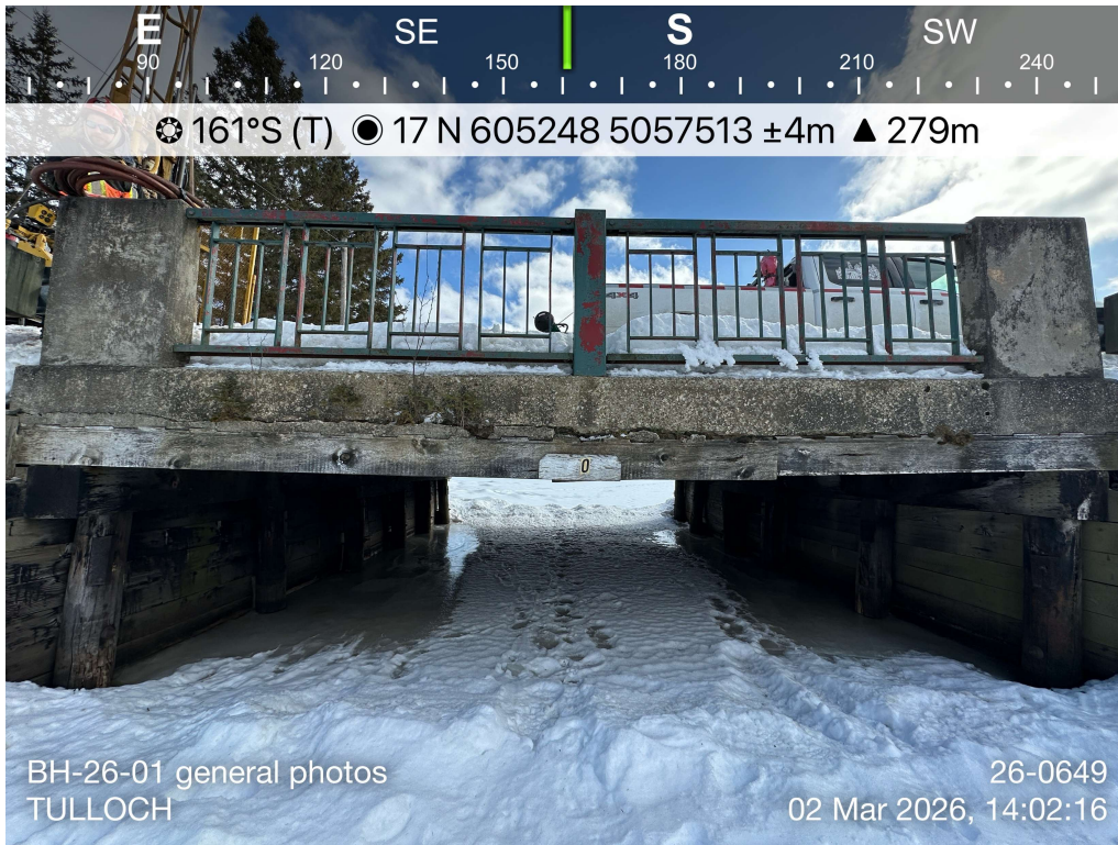
Photo 1: Existing Bridge – North Side.
