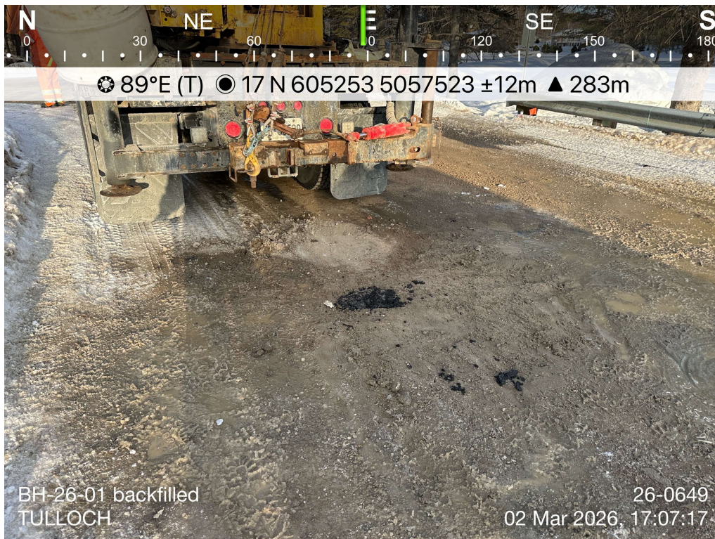
Photo 6: BH-26-01 backfilled. Photo taken facing east.
