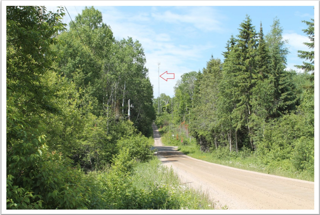
Photo 1: Profile View of Similar Tower Mast with Antenna Attachments (photo taken about 300 meters away along a municipal roadway)
