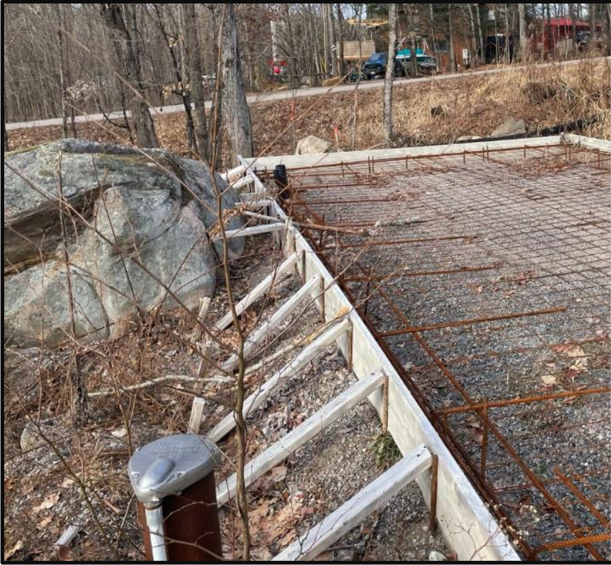
Slab form facing Magnet Road
