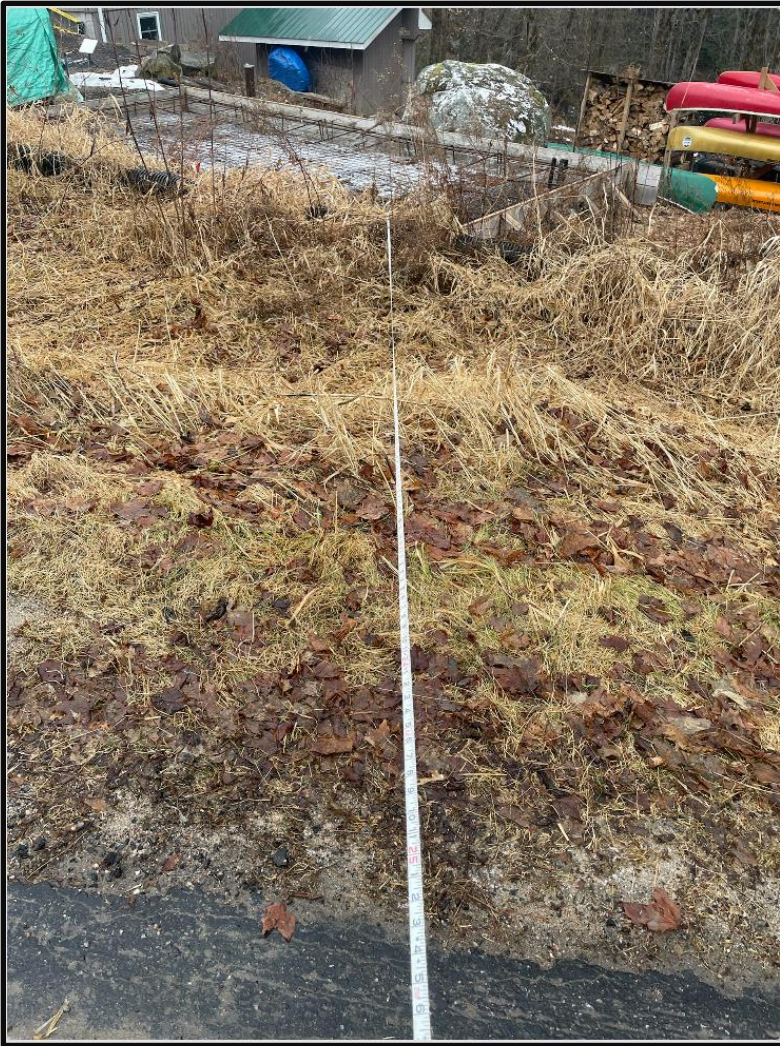
Road pavement facing property
