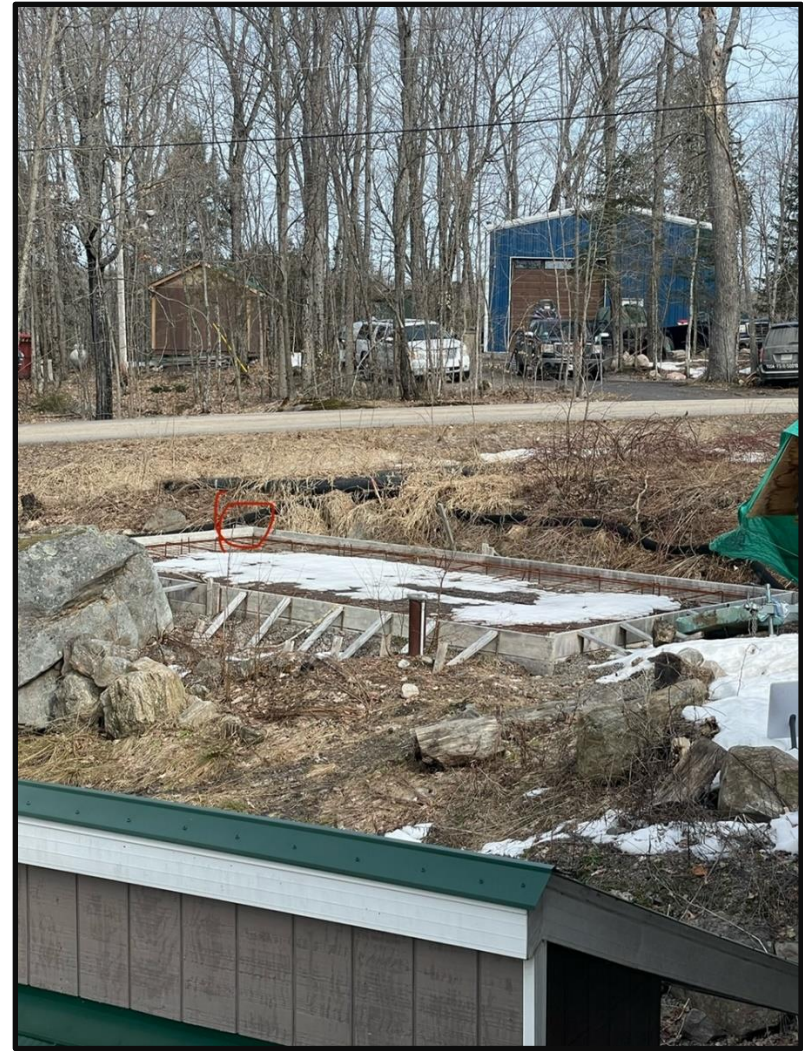
Slab Form with boulder and neighbouring detached garage
