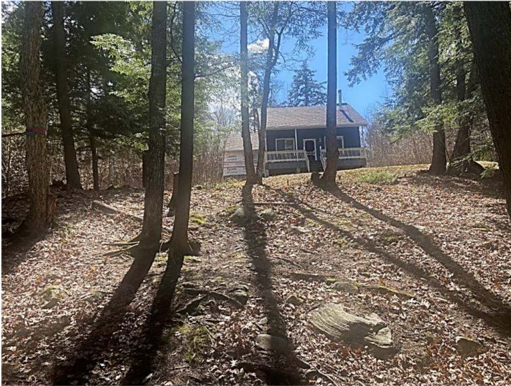
Photograph 1. View of existing cottage on proposed retained lot (April 10, 2024).
